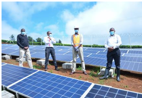
REDAVIA installer and clients in front of solar panels.
